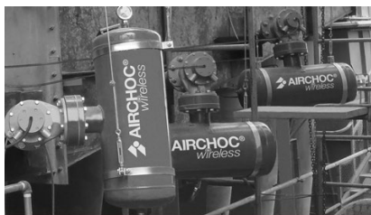
BLOCKAGE & BUILD-UP REMOVAL
