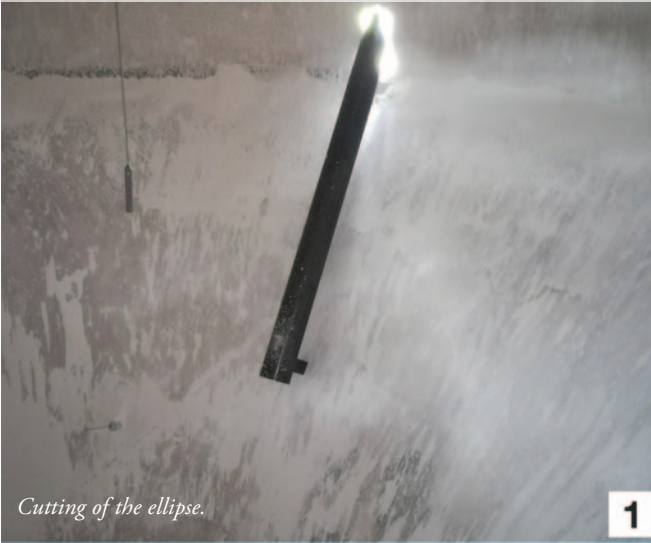
Installation by STANDARD INDUSTRIE teams of an AIRCHOC® air cannon on a sodium bicarbonate silo in order to avoid clogging of the material stored inside.
