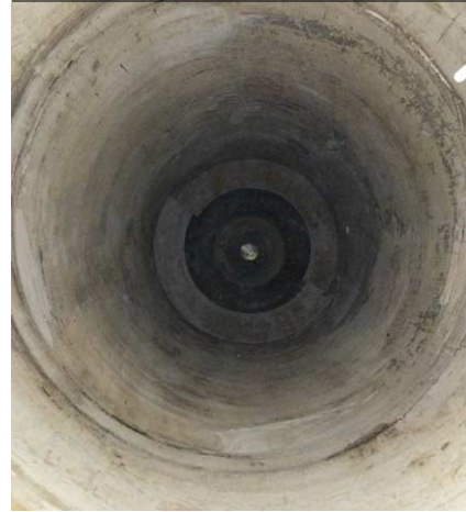
Photo 6. Bran silo that has been cleaned with the ATEX Gironet application.
