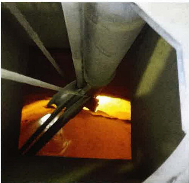
Cleaning of cement silos in South Africa.
