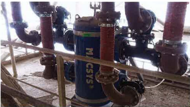
A MACSYS® Wireless that was recently installed at an Austrian cement plant.
